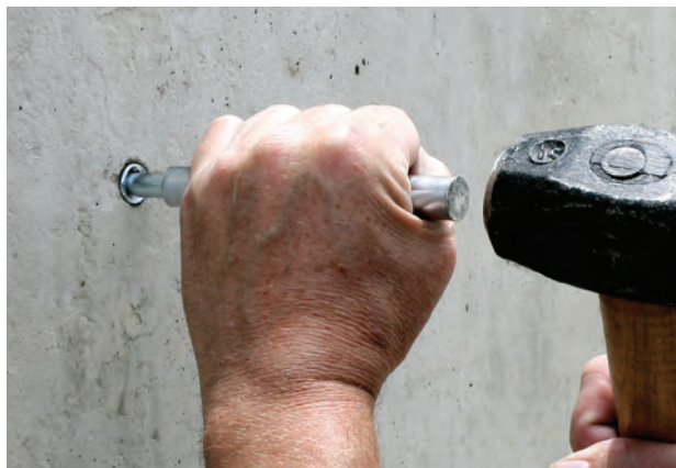
Anchor being set with hand setting tool.
