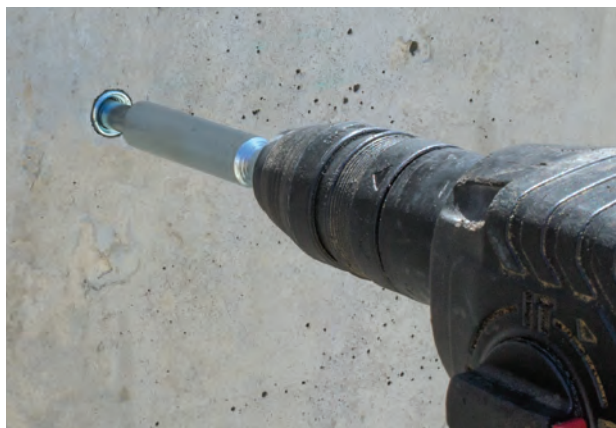
Anchor being set with SDS setting tool.
